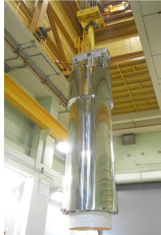
Twenty-five irradiated fuel rods from the commercial Byron Reactor being received at Idaho National Laboratory.
