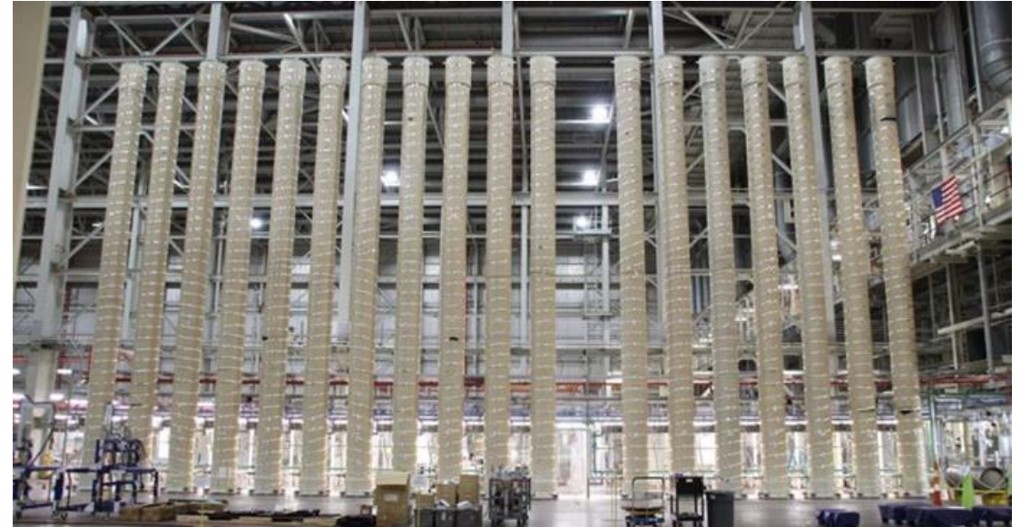
The first and only HALEU enrichment facility licensed in the U.S.
