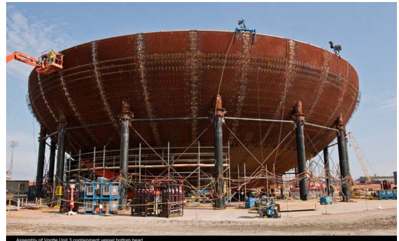
Assembly of Vogtle Unit 3 containment vessel bottom head
