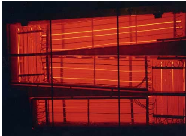
Figure 3-5. Air-Cooled Radiator in the 8-MWth MSRE in Operation. Bright yellow lines are electric heaters provided to prevent overcooling. Here they are operating because the enclosure has been opened to allow the photograph to be taken (Credit: ORNL).
