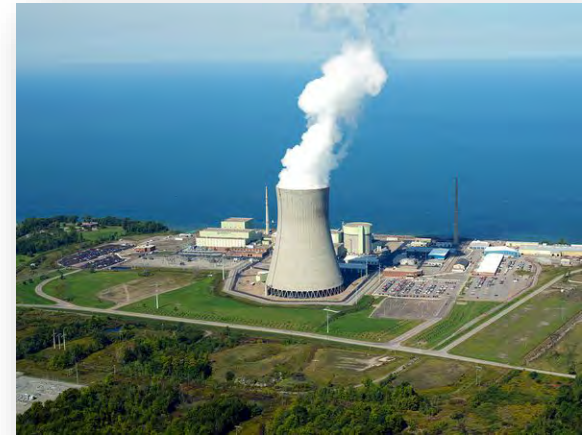
Nine Mile Point ~ Courtesy Constellation Energy
