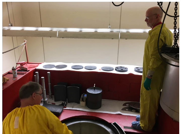
Bob Busch and Ken Carpenter dismantling the AGN-201M reactor in 2019. The fuel from the reactor (which has essentially no burnup and is thus only slightly radioactive) sits on white paper across the center of the picture. The fuel is about the same size as the barbell weights commonly found in gyms. Photo credit, Larry Wetzel.
