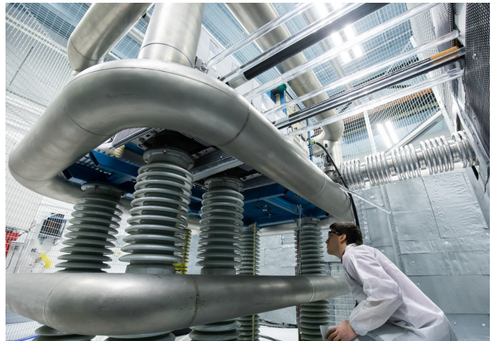
Dr. David Woodley inspecting the high voltage stack on the 400 kV ion implanter.
