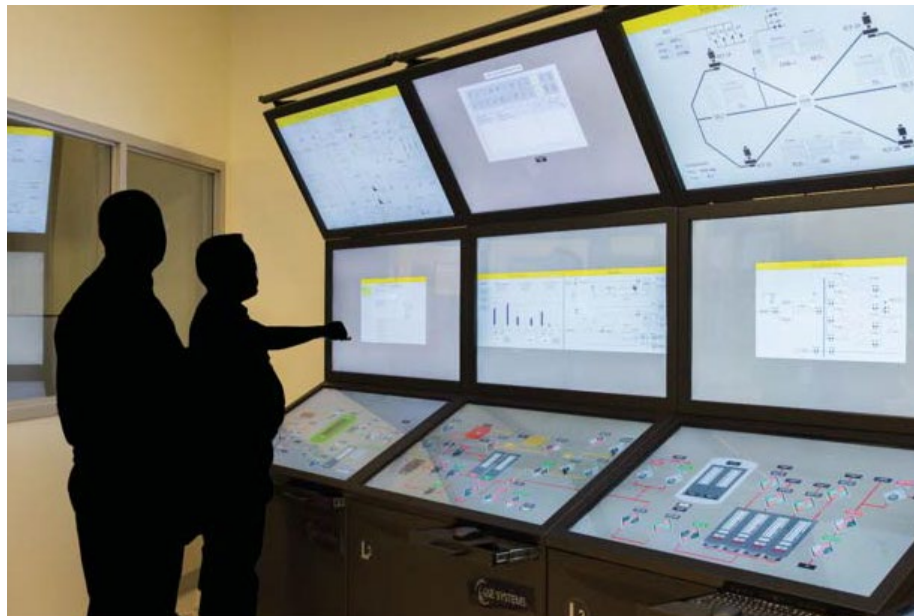
Human performance assessment with Palo Verde operators was done to simulate fault injection to gauge operator performance for PRO-AID assisted and non-PRO-AID-assisted scenarios.
