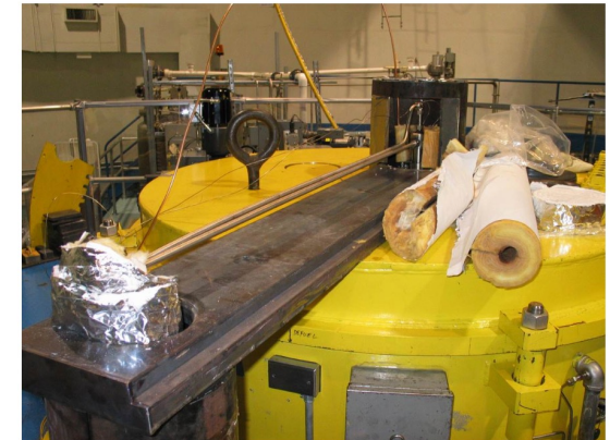
Figure A4. The ACI top head and coolant lines after facility installation in the MITR and during installation of the thermal insulation and shielding.
