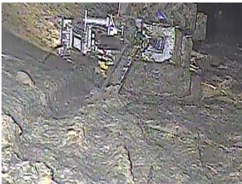
Debris created uneven surface
