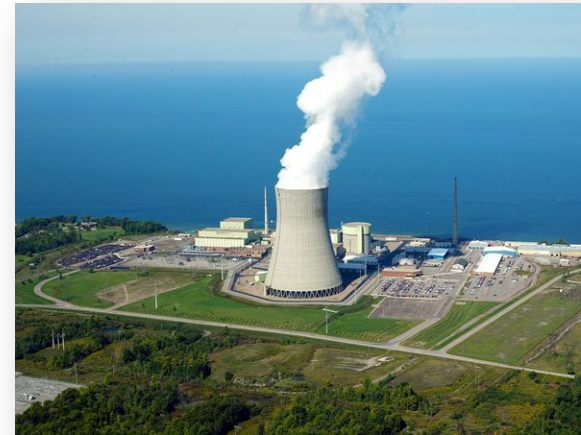
Nine Mile Point ~ Courtesy Constellation Energy
