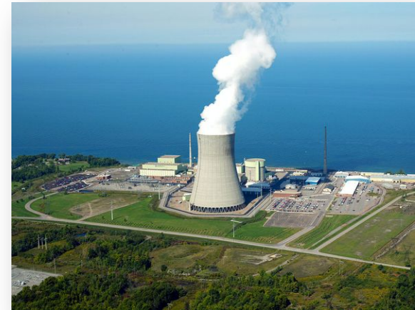
Nine Mile Point ~ Courtesy Constellation Energy
