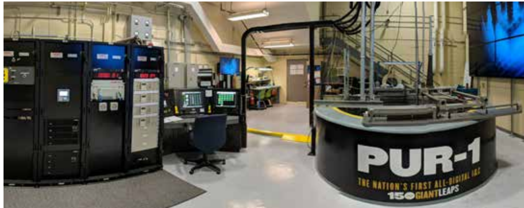
PUR-1's first-of-a-kind all-digital instrumentation and control systems upgrade.
